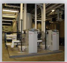
efficient water heaters tied into a vent that extended up through the building. The Lexington Plumbing team removed the old units and installed two 800,000 Btu/hr ARMOR models, stacked with two 500-gallon insulated storage tanks to provide maximum savings. With ARMOR's
